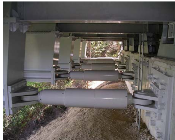
Photo 1 DAMPERS INSTALL (4A)
